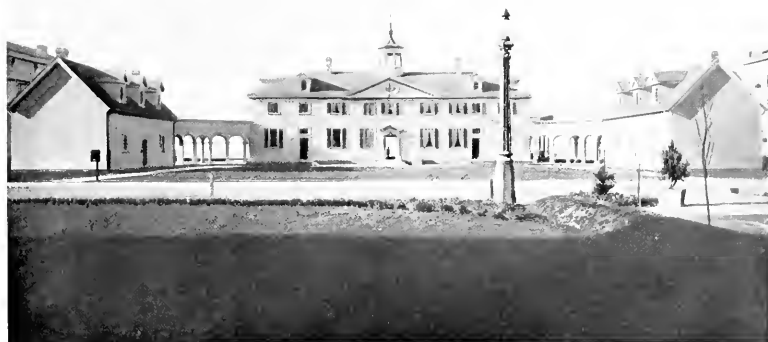
THE VIRGINIA BUILDING
